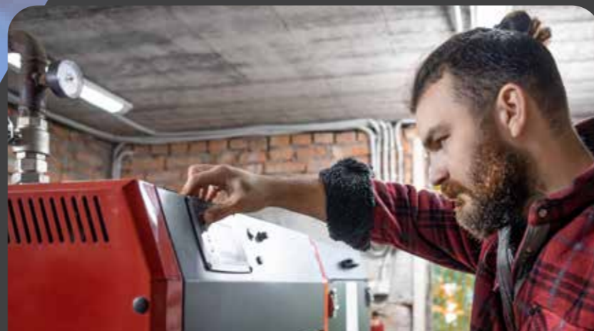
Heating and Ventilation Services
