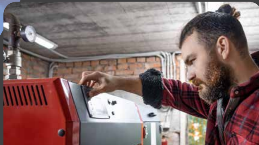
Heating and Ventilation Services
